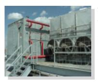
A large New England bakery produces the rolls used to make deli sandwiches for a chain of fast food outlet stores. In the production process, the bakery uses a 300ton open recirculating cooling water system to chill the plant's ammonia-based
